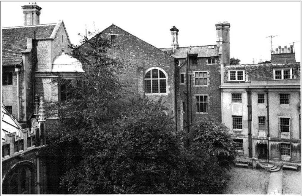
FIGURE 5. PROTRUSION OF REAR OF INDIAN INSTITUTE
