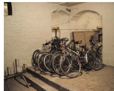
The Crypt before refurbishment
