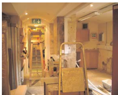
The old Swift Room undergoing refurbishment
